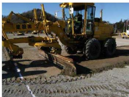
Removal of topsoil at a school
