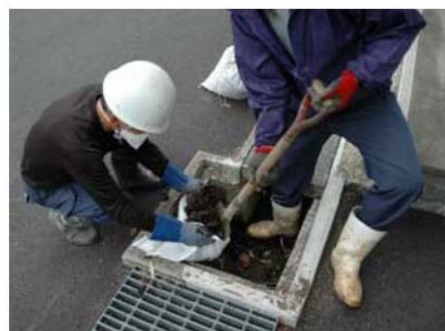
Removal of sediment from gutters
