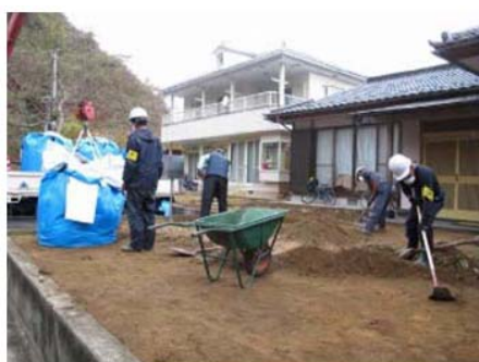
Removal of topsoil
